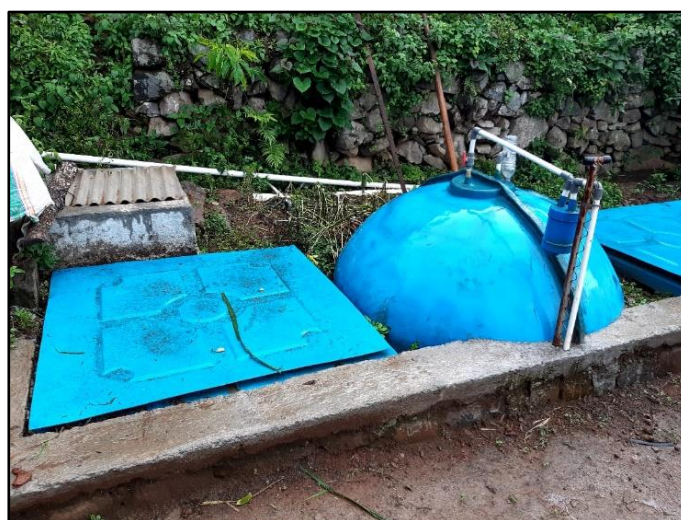
Figure 5. Biogas digester made of polyethylene applied by Banyudono dairy farmers (source: documentation of authors, 2019)
