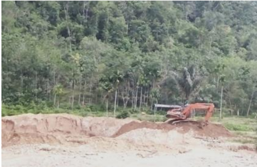
Gambar 5. The use of excavator in the excavation process.
