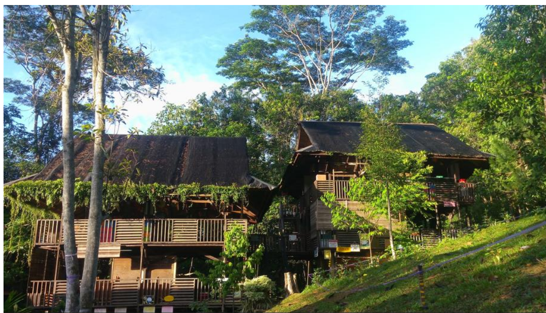
Figure 1. Classroom building at Sekolah Alam Balikpapan with nipa thatched roof covered with netting
