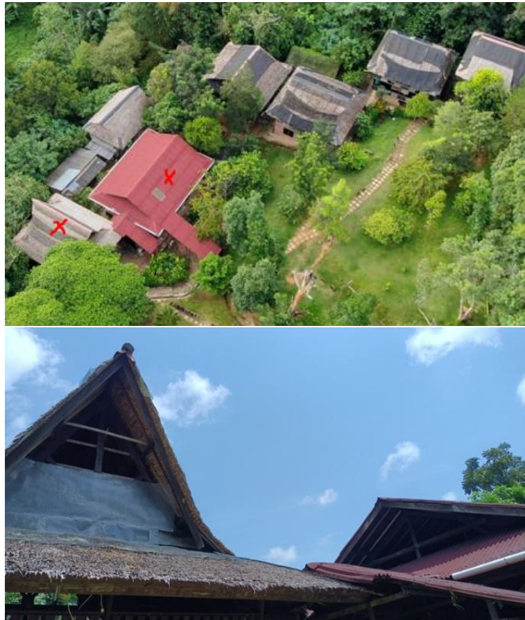
Figure 2. Aerial photo of Sekolah Alam Balikpapan, bitumen roofing (red) and nipa roofing (brown)
